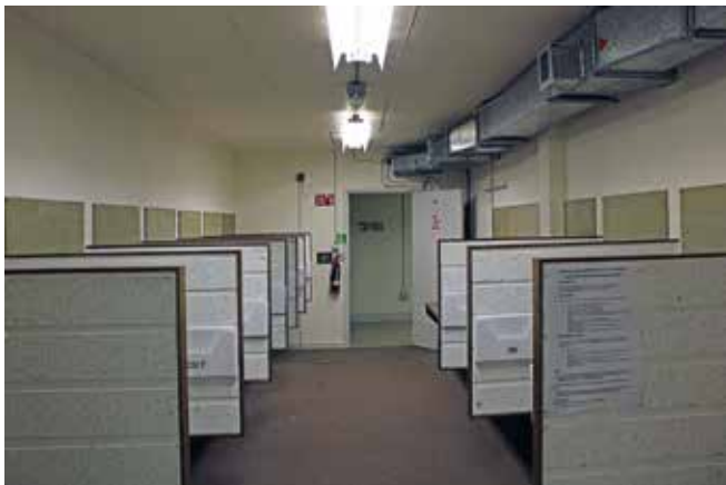
Communications centre in 2018, now stripped of loose furnishings and wall maps
